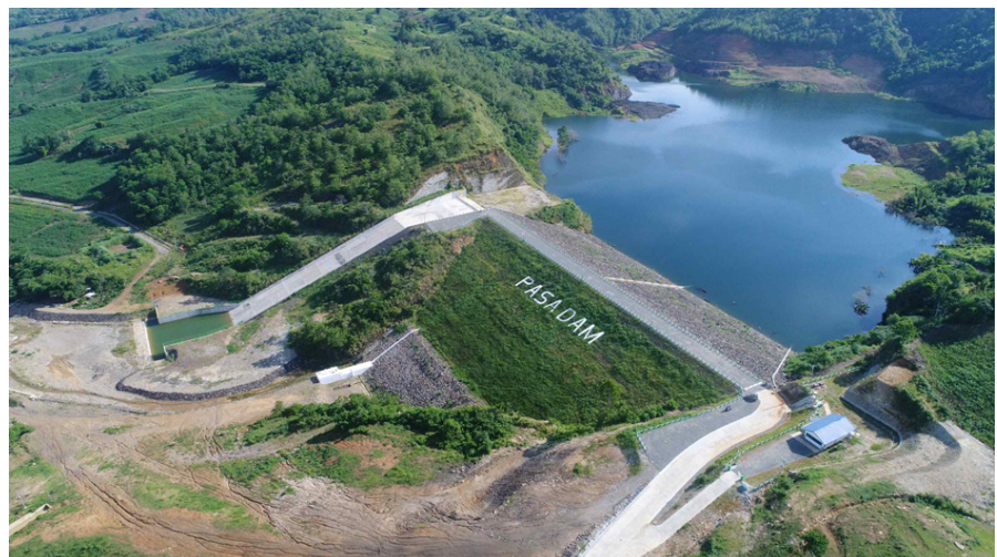
FIGURE 4. PHOTOGRAPH OF THE COMPLETED PASA DAM
